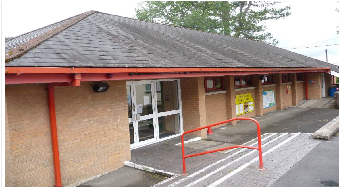
External view of the hall and canteen building
